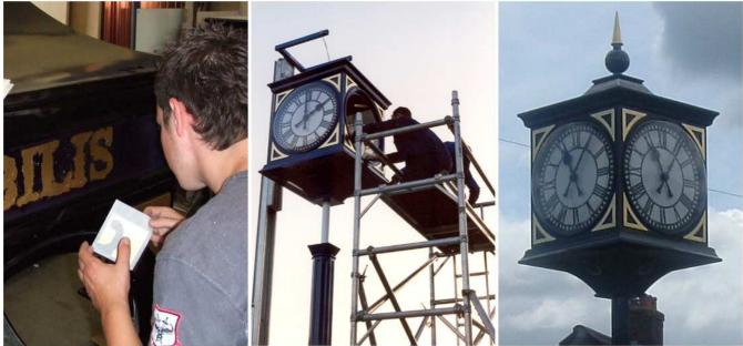
Top: St Clears Bottom left: Town name being applied in gold leaf Bottom middle: Dial box being lowered on to the pillar Bottom right: Close up of a dial box
